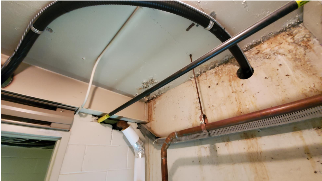
Figure 5: Underside of Podium slab exhibiting evidence of excessive water infiltration through a crack and at the cold-joint between the slab and basement wall.
