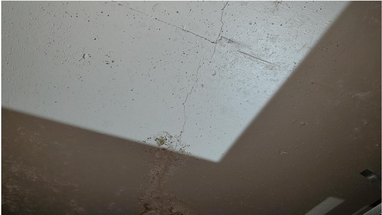
Figure 3: Typical shrinkage crack at underside of slab without any evidence of water infiltration.
