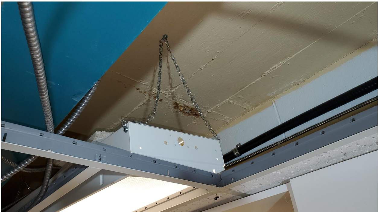
Figure 4: Underside of Podium slab exhibiting evidence of minor water infiltration through a crack.
