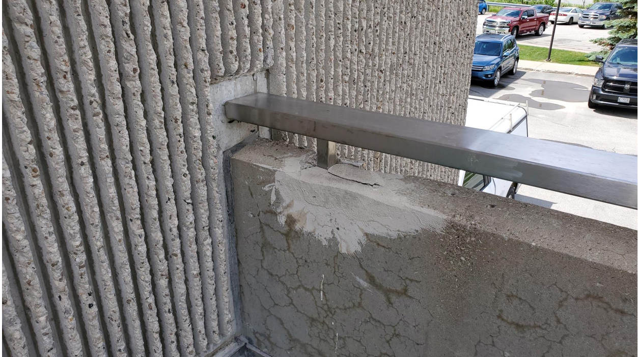
Figure 19: Map-cracking on concrete surface and previous repairs / delamination at steel guard connection.
