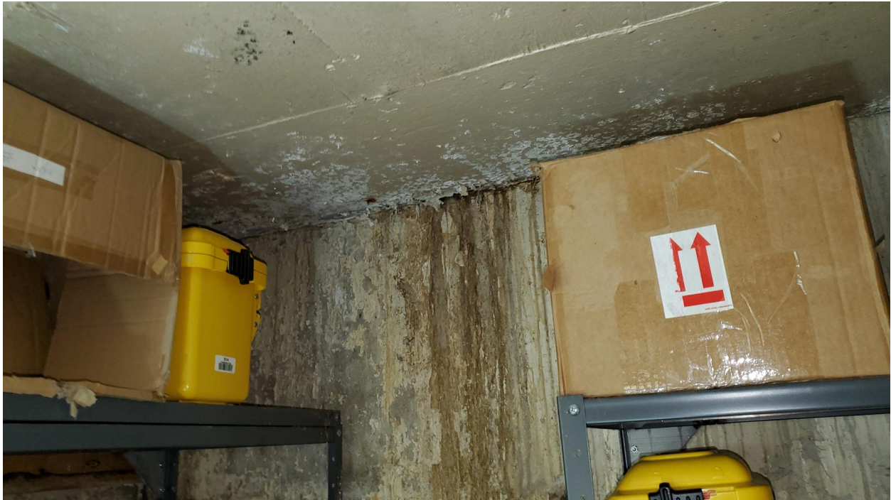
Figure 9: Cold-joint between the concrete slab and basement wall exhibiting evidence of excessive water infiltration.
