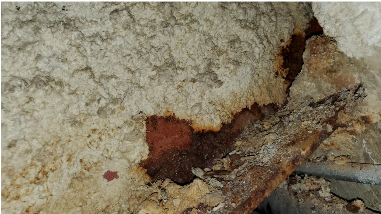
Figure 16: De-bonded spray-applied fireproofing and minor section loss of steel beam at basement wall.
