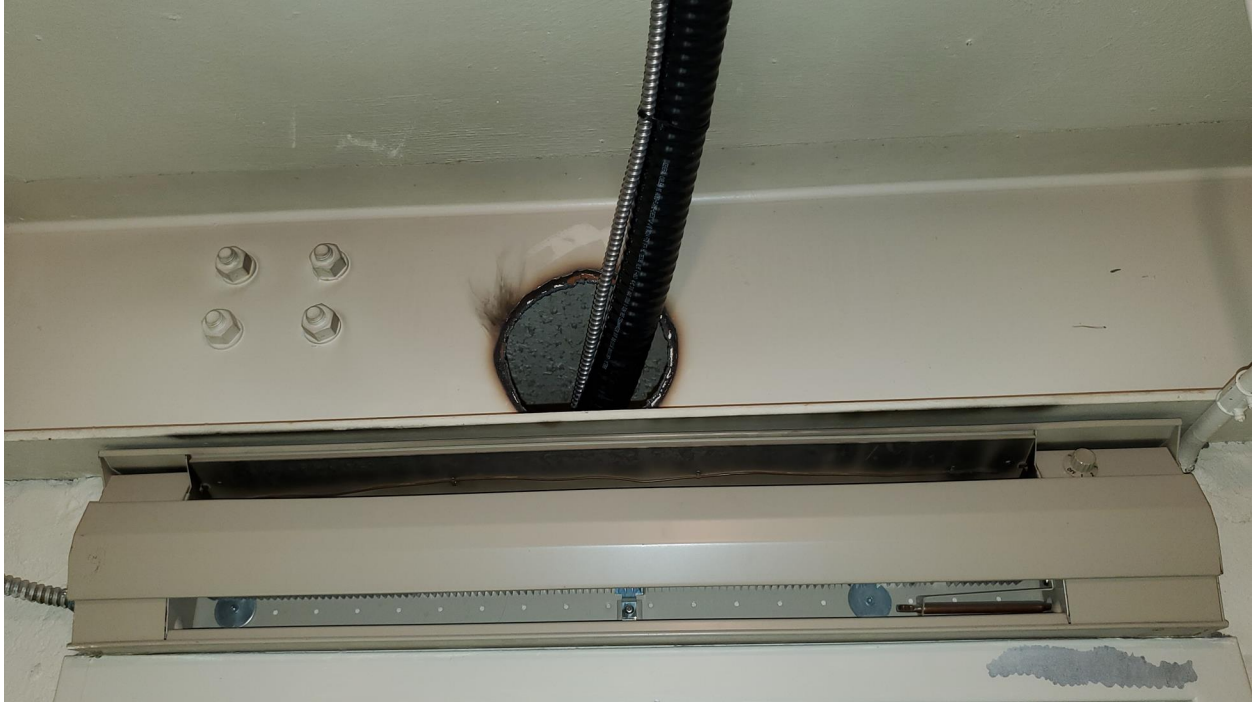
Figure 17: Unreinforced opening cut through existing beam web on gridline 1, between J and K.
