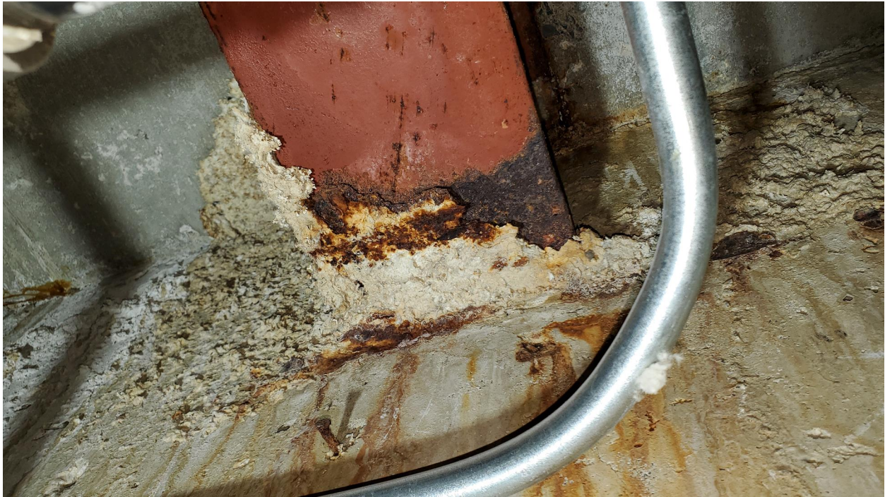
Figure 15: De-bonded spray-applied fireproofing and minor section loss of steel beam at basement wall.
