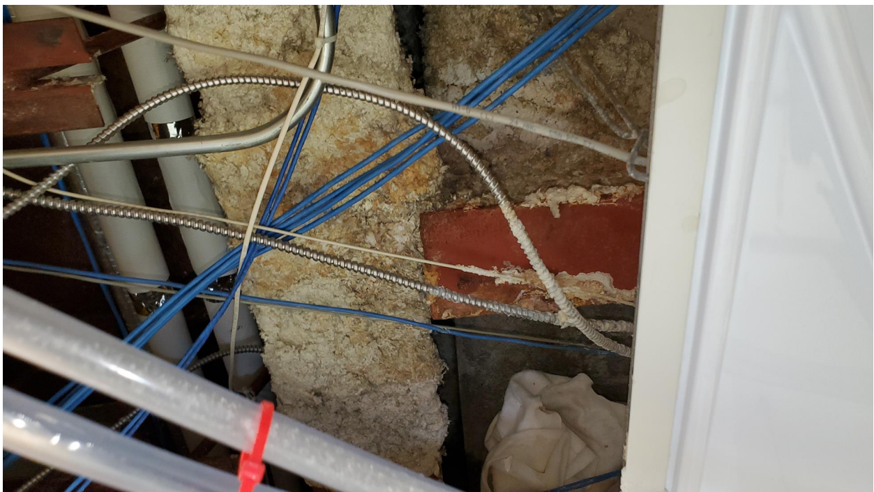
Figure 14: Spray-applied fireproofing on steel beam exhibiting minor exposure to water.
