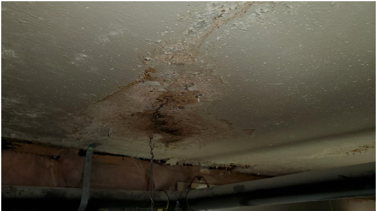
Figure 6: Underside of Podium slab exhibiting evidence of excessive water infiltration through a crack.
