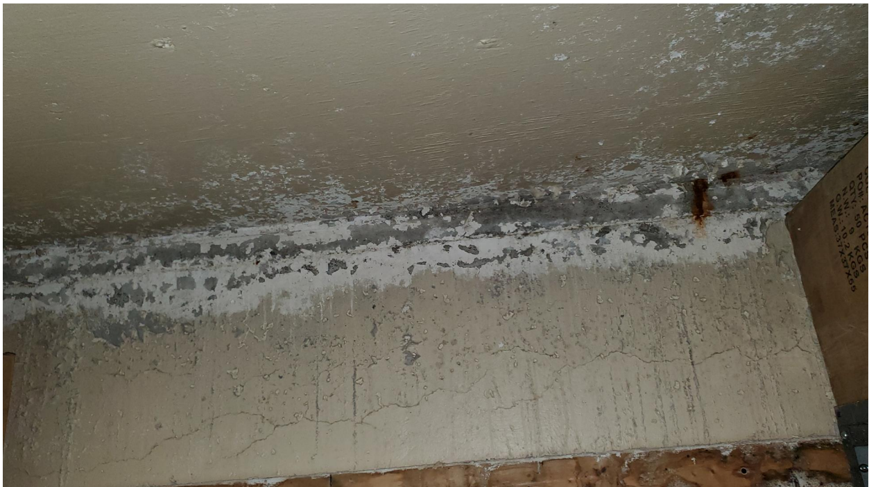
Figure 8: Cold-joint between the concrete slab and basement wall exhibiting evidence of excessive water infiltration.
