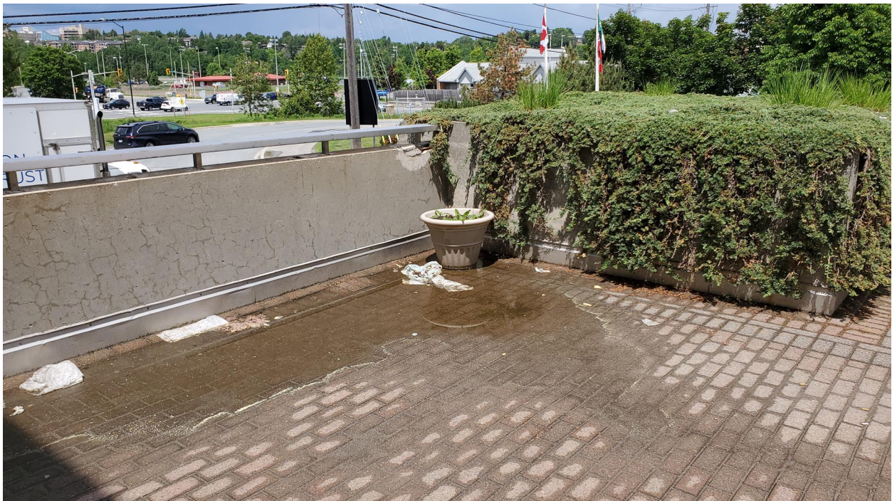
Figure 18: Standing water at west side of Podium.
