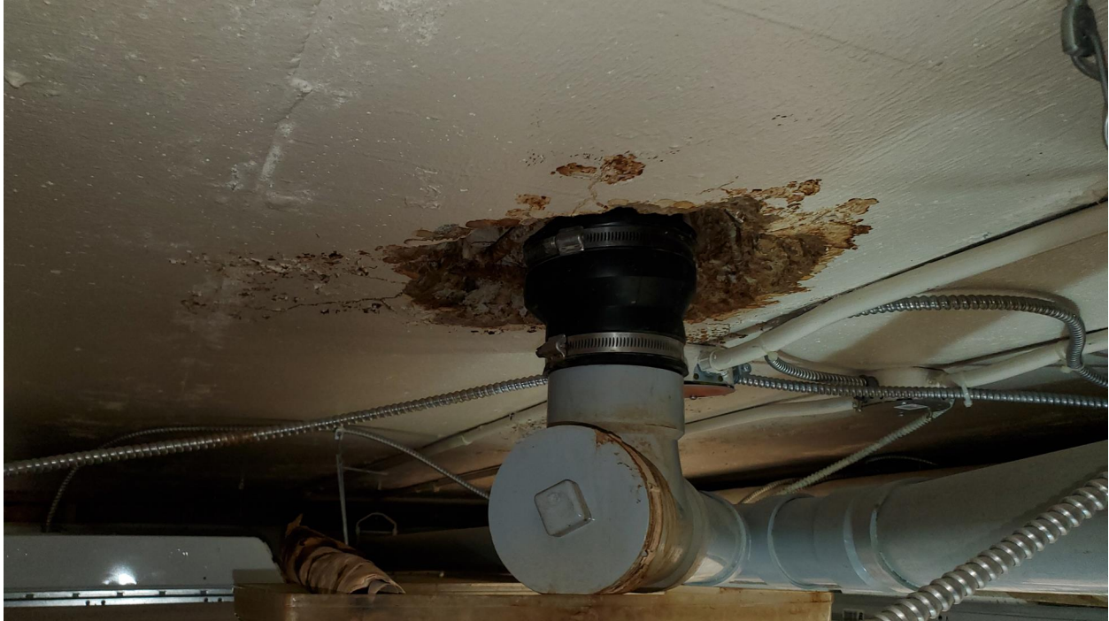
Figure 7: Underside of Podium slab exhibiting evidence of excessive water infiltration at a drain.
