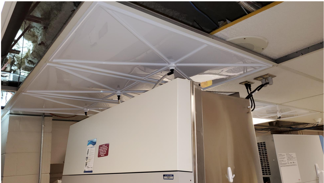
Figure 10: Ceiling catchment system installed in the Laboratory.
