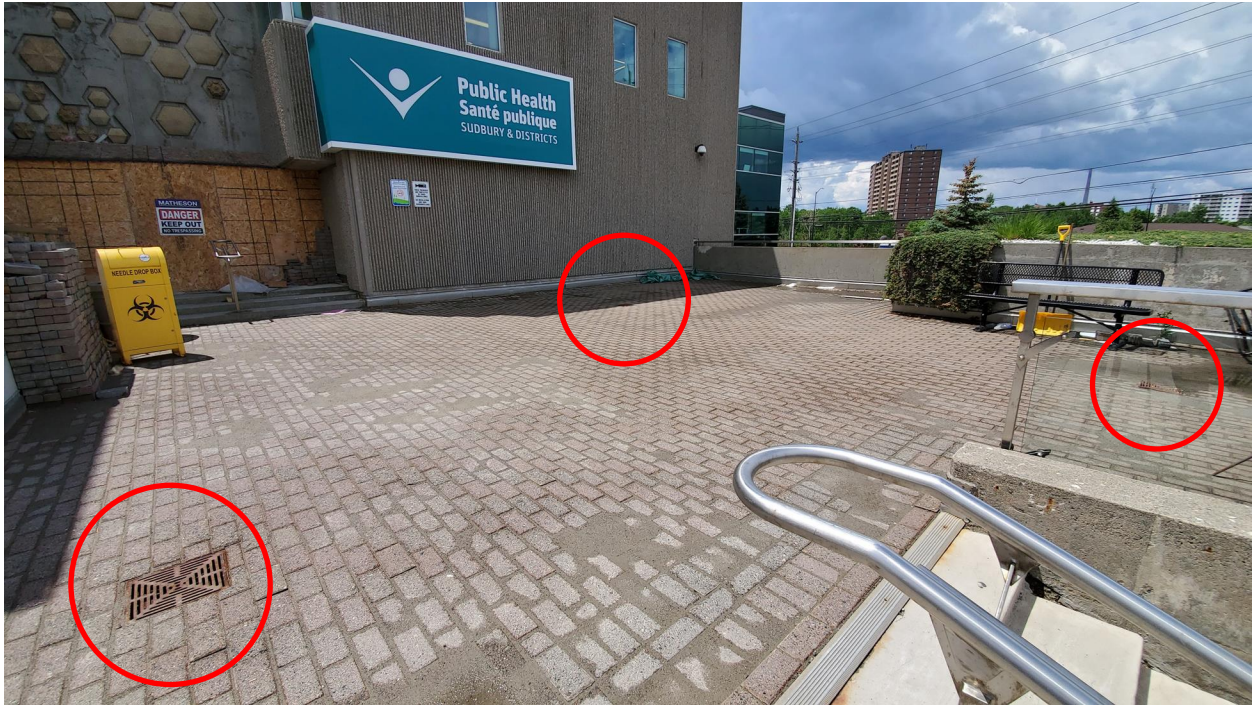
Figure 1: Podium surface looking southwest. Drain locations noted.
