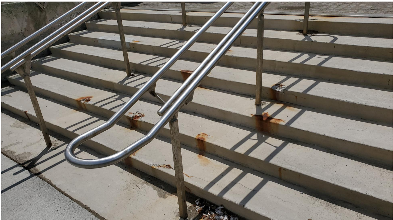
Figure 12: Lower stair. Note rust stains, cracks, and delaminated concrete.
