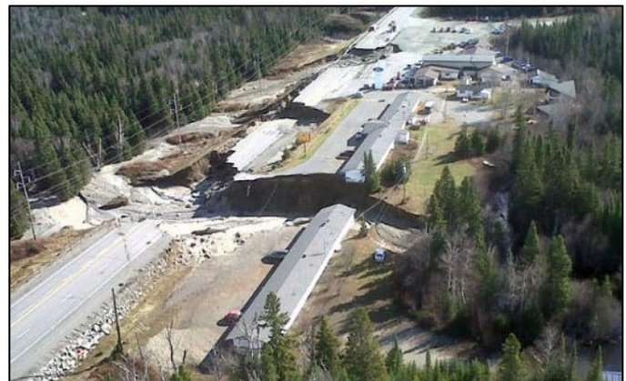
Figure 8: Torrential rains cause wash outs of Highway 17 at Wawa, Ontario, in October 2012; the township declares a state of emergency.
